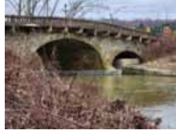
Oldest stone arch bridge in WV!
